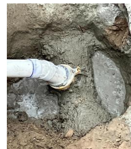
This is the new drain line going under the yellow gas line, abandon gas line and 2003 water line
