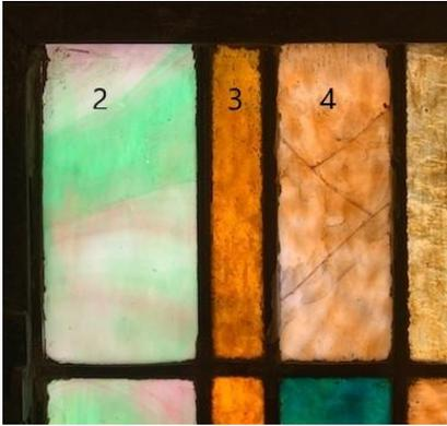
If the cracks in a pane cannot be repaired, the pane will need to be replaced. The replacement glass will come from three crates of custom-made glass that will be procured as part of this project to match the primary colors of glass in our windows. After procuring the custom glass, we will have an adequate supply of replacement glass to use for future restoration projects.
