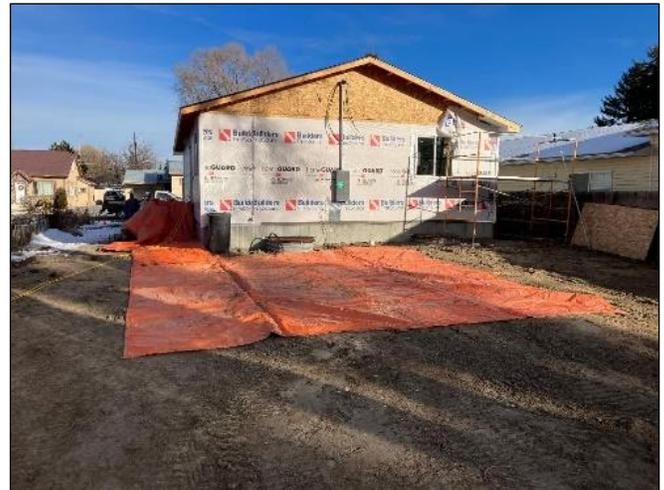
In the backyard of the Habitat house, the sewer and freshwater connections have been made and buried. Preparations are made for a 20' x 20' concrete pad and sidewalk going to the house. Orange tarp keeps the dirt dry and warm before the concrete. The concrete pour will include the slab, two outside stairs and replacing the front sidewalk along 18th St.
