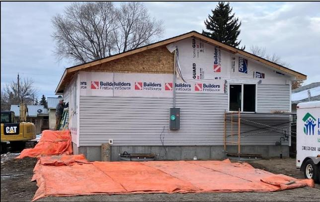
In the front the new sidewalk and front steps are poured and curing under the orange blankets. The blankets should be able to come off by Friday.
