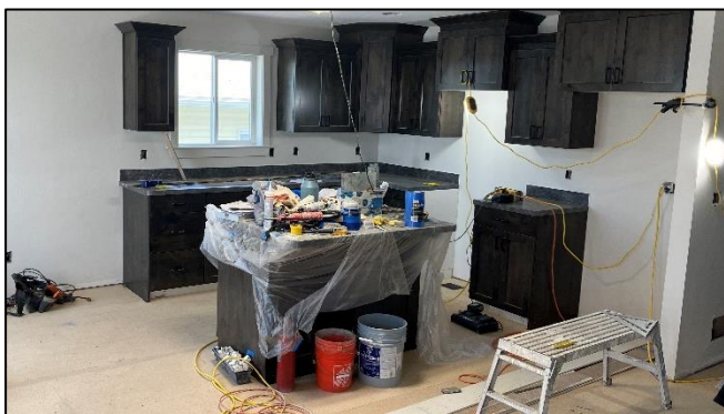
Installing the flooring in the kitchen and the
