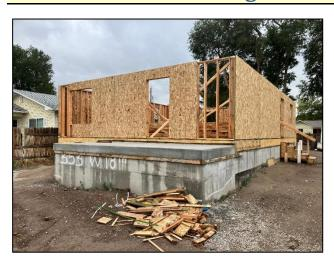
The Habitat house is progressing. The exterior walls that were made at St Paul's are in place and most have the chipboard exterior sheath attach. The interior walls are stacked inside waiting to be stood up and secured to the exterior walls. Soon we will see the roof trusses in place.
